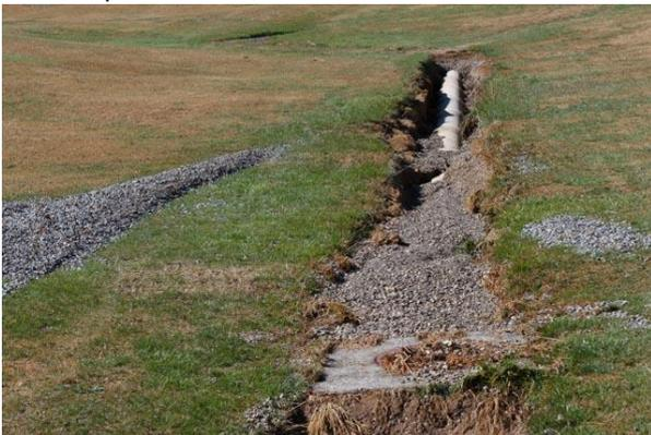
The drain in the hazard in front of the 2<sup>nd</sup> tee blocked up, the water overflowed and then ran down the 1<sup>st</sup> fairway washing out a lot of the drainage chip in the centre of the fairway and removed a lot of the sand from our new drains. Also the drains to the right of the 1<sup>st</sup> fairway blocked up with water again flowing over the top and leaving a lot of debris behind.
